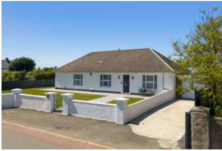
Front Parking Area & Garden
