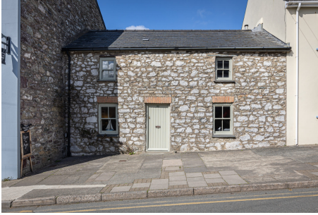
Parking Area & Entrance Door
