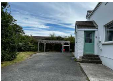
House Entrance & Parking Area
