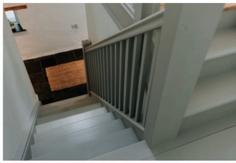
Stair to FF Bedrooms
