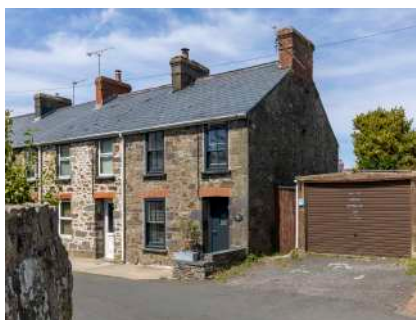
Entrance Door & Street
