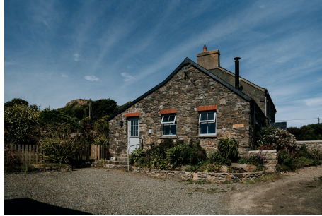
Parking Area & Entrance
